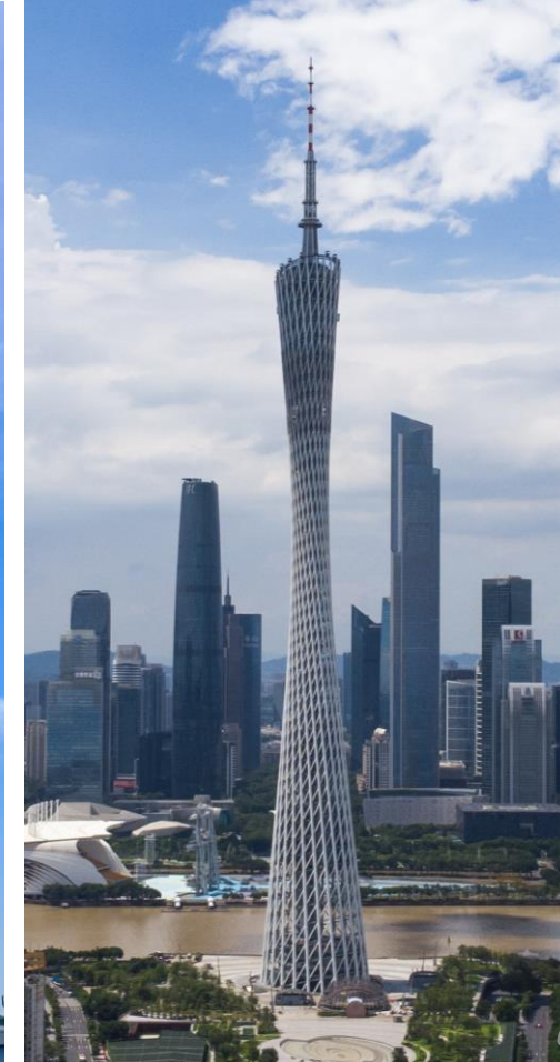
Self-supporting hyperboloid lattice tower of Guangzhou , China
