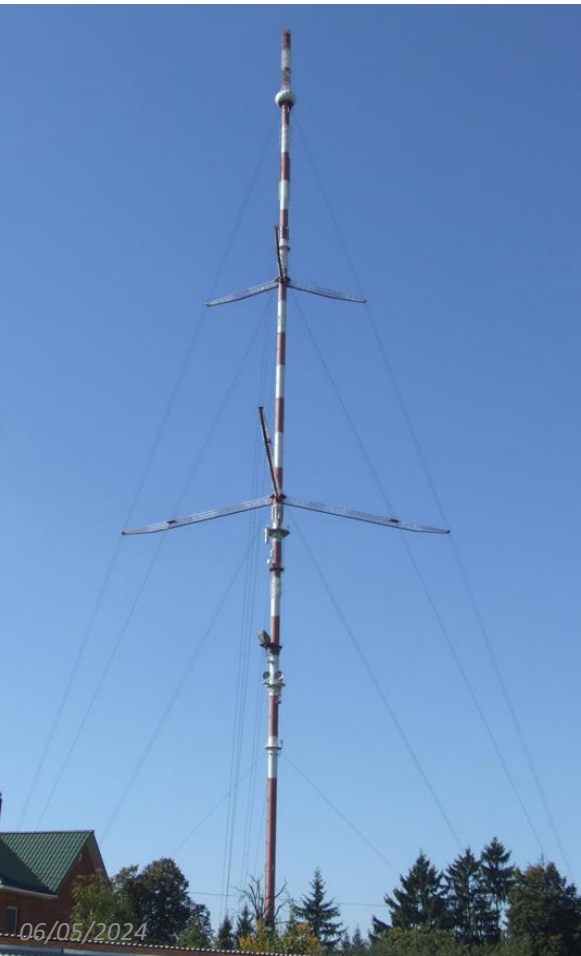
Guyed steel tube mast of STBS Vinnytsia , Ukraine
