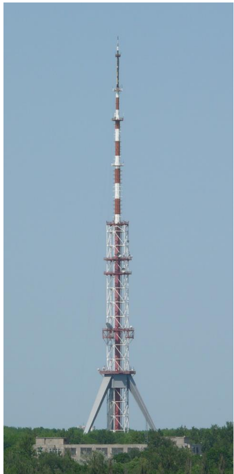
Lattice steel hexagonal tower of STBS Kharkiv , Ukraine
