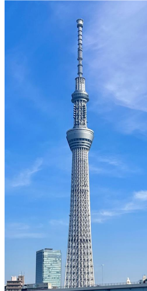
Reinforced concrete / lattice broadcasting tower of Tokyo , Japan
